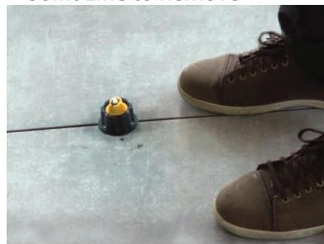
7. Unlock Yellow Cap, Discard the Screw and Reuse Cap
